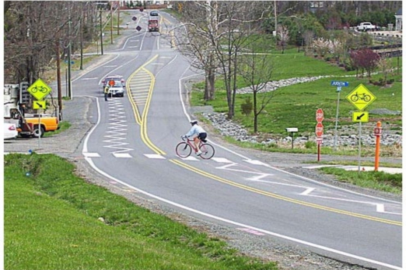
Figure 10. Zig-zag Markings at Belmont Ridge Road
